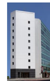
A92 KDX Akihabara Building
