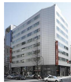
A40 Toranomon Toyo Building
