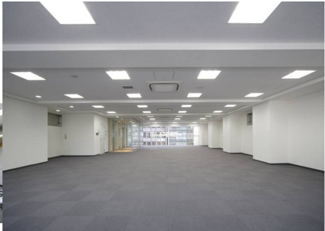
After renovation—Typical floor
