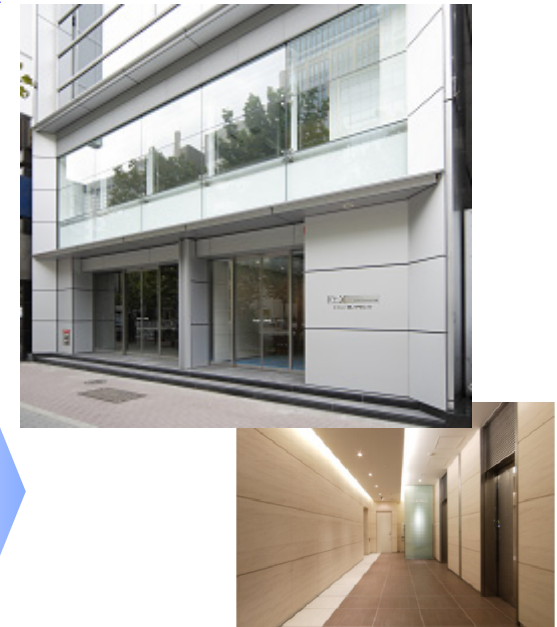
Entrance hall after renovation
