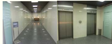
<KDX Kayabacho Bldg. before renovation>
