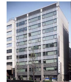
KDX Nihonbashi 313 Building (Seismic review by NIHON SEKKEI, INC.)
