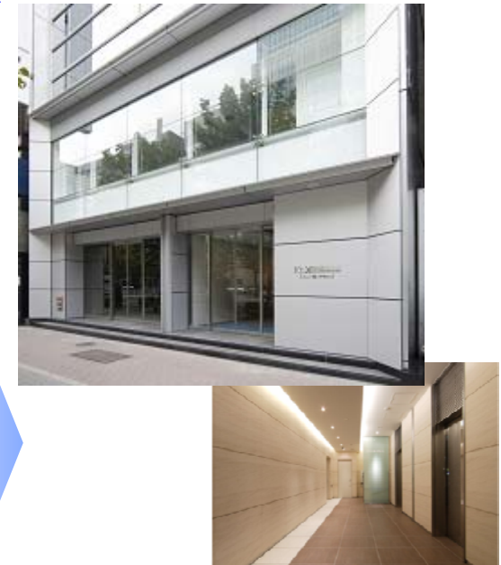
Entrance hall after renovation
