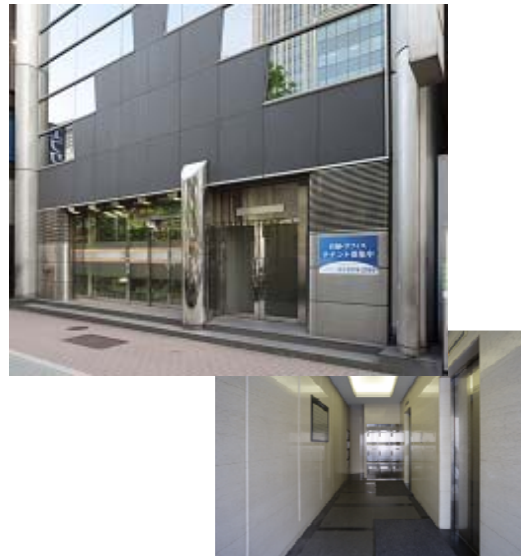
Entrance hall before renovation
