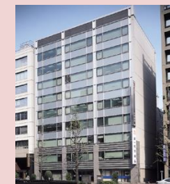
KDX Nihonbashi 313 Building
