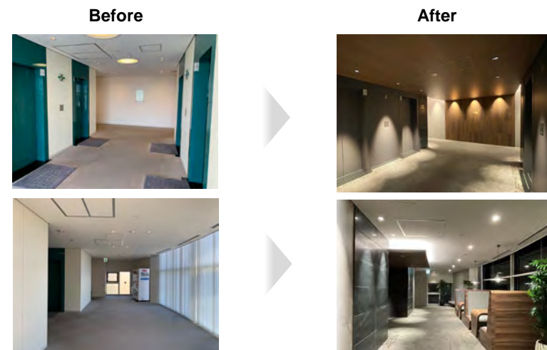
Renewal of common areas on the 4th and 7th floors of the KDX Chofu Building (improved tenant satisfaction)
