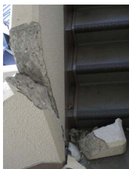
External stairs handrail (4F apart)
