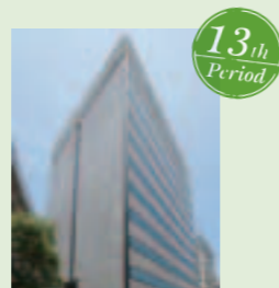
A-73 KDX Hakozaki Building Location: Chuo-ku, Tokyo Gross Floor Area: 6,332.48 m 2 Acquisition Price: 2,710 million yen Acquisition Date: July 22, 2011
