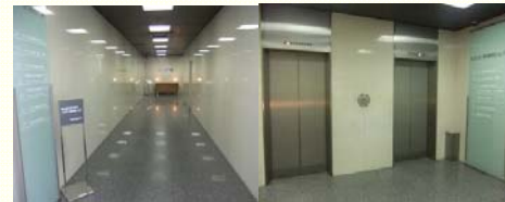
<KDX Kayabacho Bldg. before renovation>
