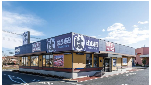
Constructed restaurant building at Unicus Ina
