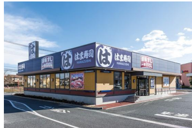
Newly constructed restaurant building
