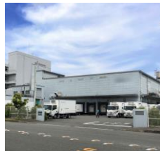
Oppama Distribution Center
