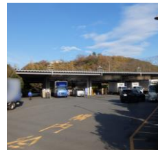
Yokohama Kamigo Distribution Center
