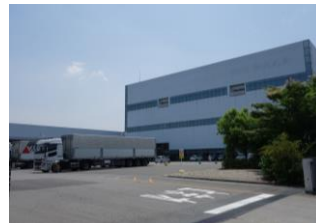
Gyoda Distribution Center
