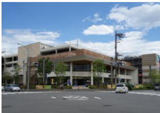
Apita Terrace Yokohama Tsunashima
