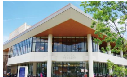
Apita Terrace Yokohama Tsunashima Power generation capacity: 25.26 kW
