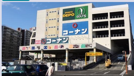
Home Center Kohnan Sunadabashi Location: Nagoya, Aichi
