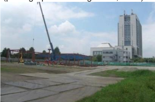
2. Construction continues... (photographed on August 22, 2015)
