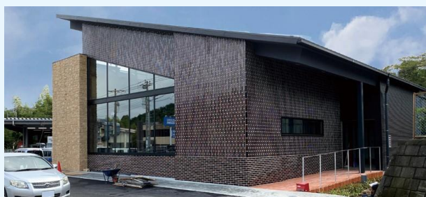
The newly built Restaurant Building
